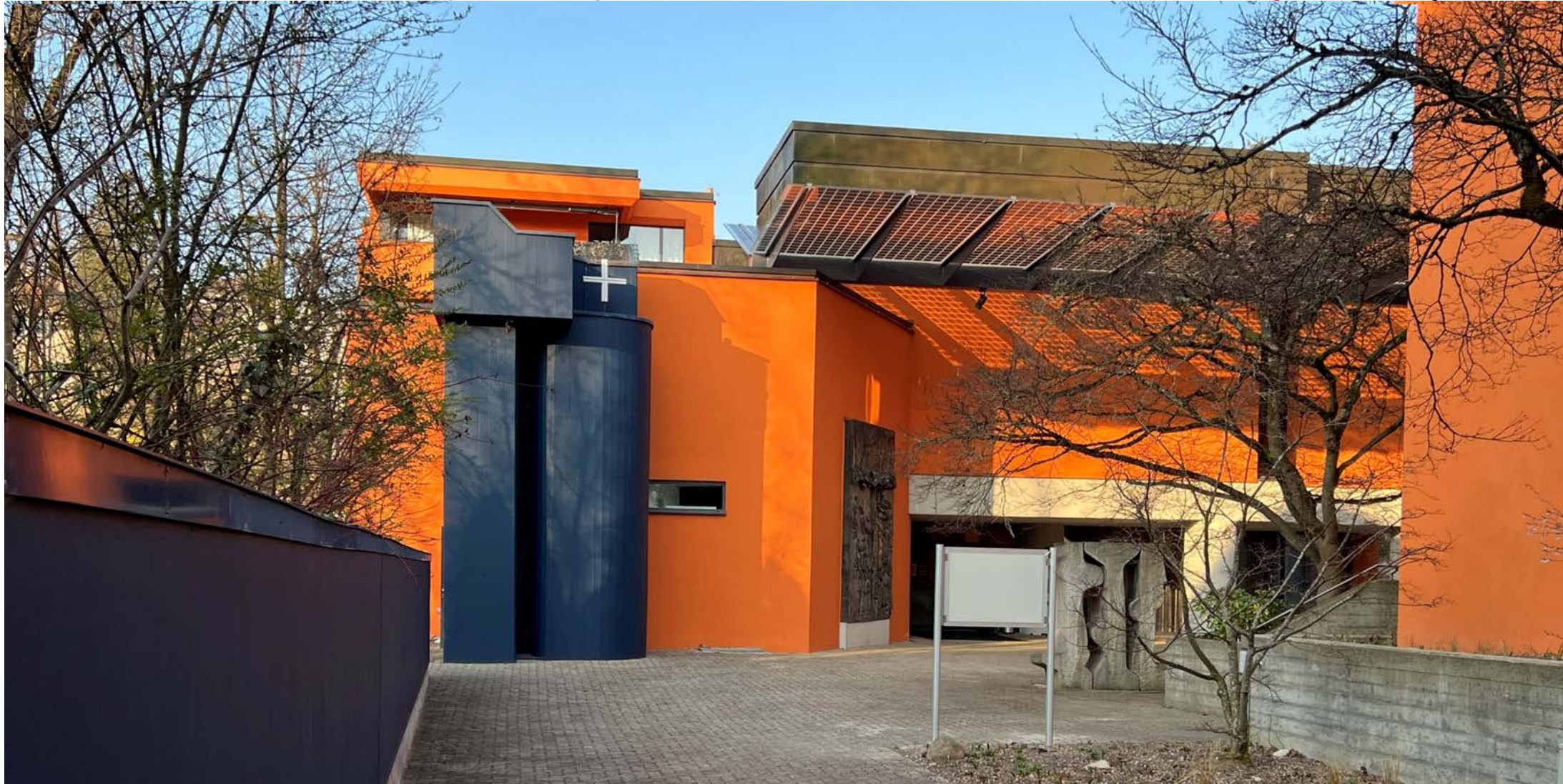
catholic parish center Heilig Geist, Zürich-Höngg, built 1973, renovated 2018 - 2020, Minergie
