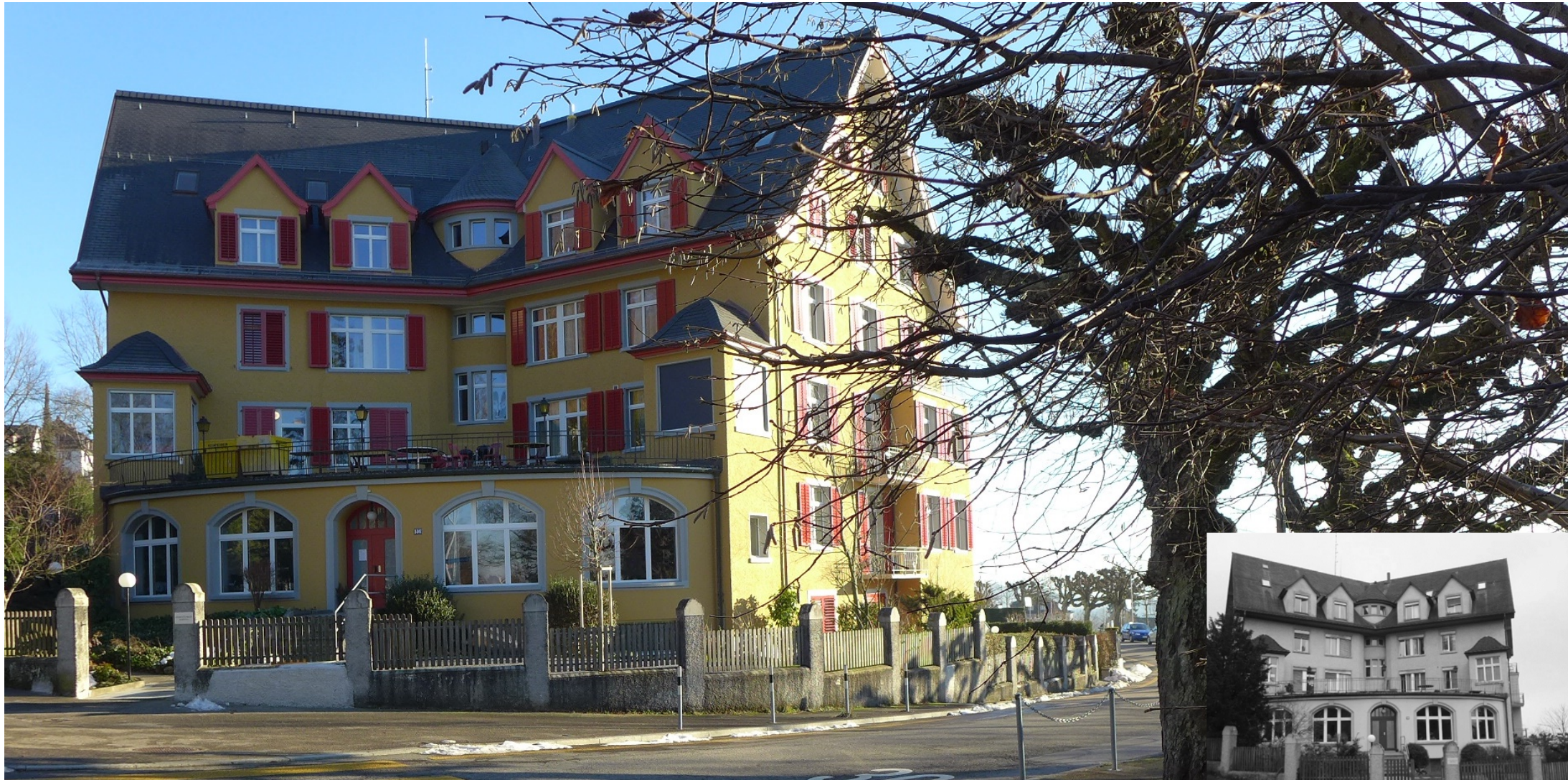
student boarding house Justinus, Zürich-Fluntern, built 1907, classified, renovated 2018, Minergie
